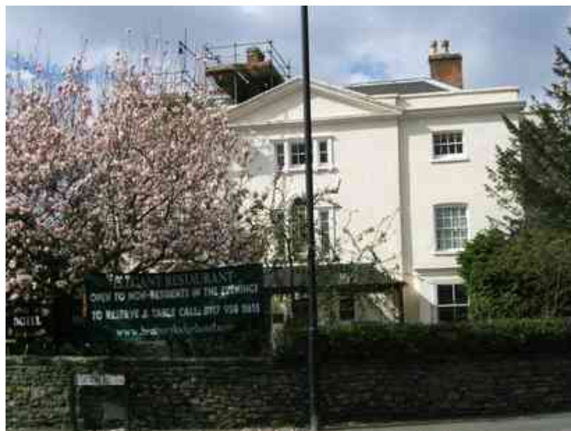
View from Station Road.
