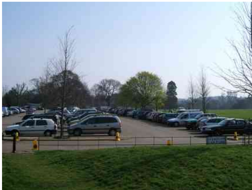
View of new car park looking towards Blaise Castle House and Conservation Area.
